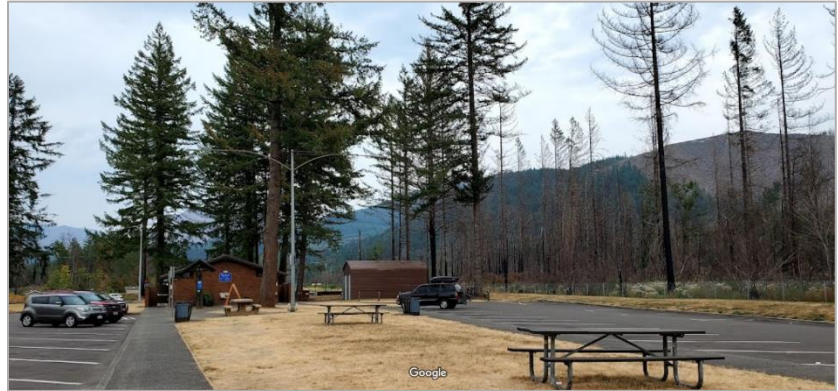
Figure 5—Maples Rest Area
